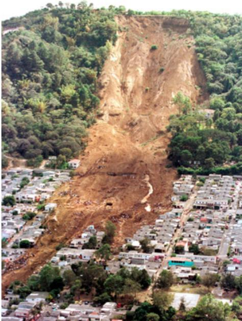
**Figure 12.29** A slope gives way in a suburb of San Salvador after the January 2001 earthquake offshore of El Salvador. This is one of hundreds of slope failures resulting from the earthquake. *Source: U. S. Geological Survey (2001) Public Domain*
