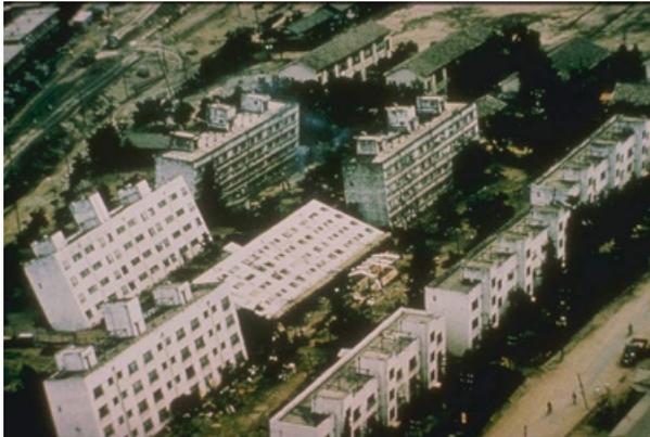
**Figure 12.26** Collapsed apartment buildings in the Niigata area of Japan. The material beneath the buildings was liquefied by the 1964 earthquake. *Source: DOC/NOAA/NESDIS/NCEI (1964) Public Domain*
