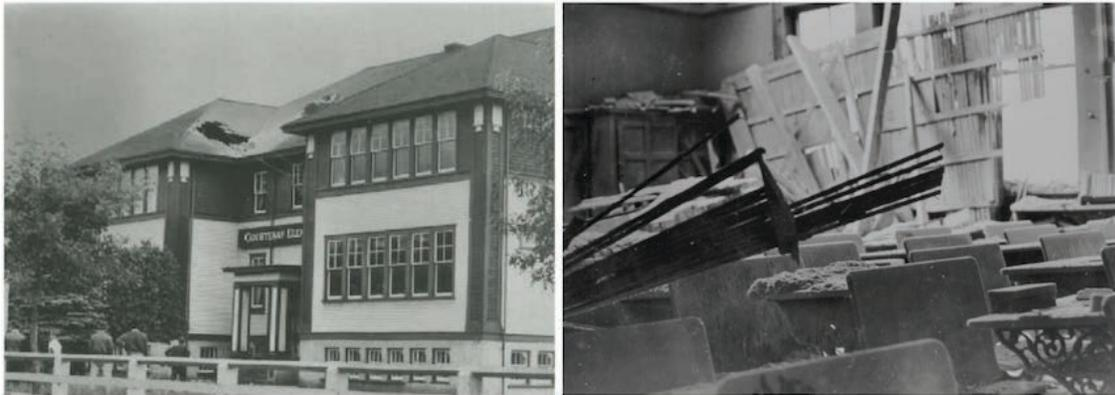
**Figure 12.2** Damage to an elementary school in Courtenay, British Columbia after a magnitude 7.3 earthquake on Sunday, June 23, 1946. Left: A hole left after the chimney collapsed through the roof. Right: Damage inside the school. In addition to damaging structures, the earthquake triggered numerous slope failures. *Source: Photographs courtesy of Earthquakes Canada. See Appendix C for image sources and terms of use.*
