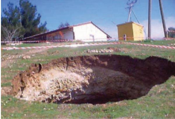
**Figure 8.10** Sinkhole downstream of the Mosul Dam in Iraq. The sinkhole is a result of dissolution of gypsum and anhydrite layers. *Source: U. S. Army Corps of Engineers (2007) Public Domain*
