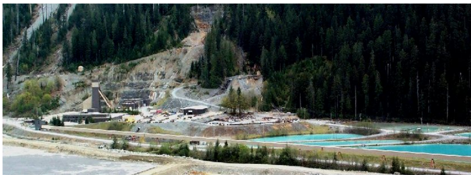
Figure 18.13 The tailings pond (lower left) at Myra Falls Mine with settling ponds (right) for processing water from the concentrator. [SE]
