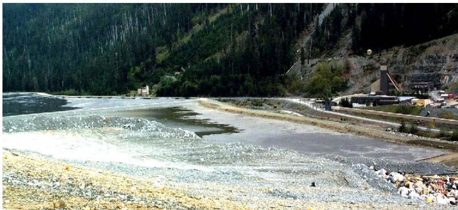
Figure 18.12 The tailings pond at the Myra Falls Mine on Vancouver Island. The dry rock in the middle of the image is waste rock. The structure on the right is the headframe for the mine shaft. Myra Creek flows between the tailings pond and the headframe. [SE]
