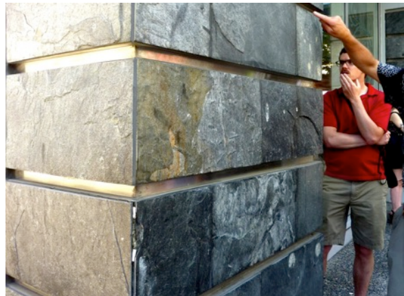
Figure 18.17 Slate used as a facing material on a concrete building column in Vancouver [SE]
